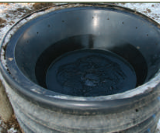
Holes in the drain-back water bowl slowly drain the water back into the wet well to avoid freezing.
