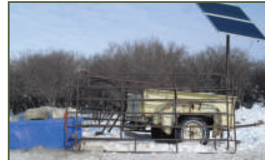
Winter Water System. Between the trailer and trough is the wet well with a submersible pump, which is powered by solar panels. The water level is regulated by a float located inside the insulated trough. This water system has been trouble free, the only maintenance is when temperatures are below -25 C they may need to tap through the ice in the drinking tubes. The ground around the well has been built up and slanted away from the well to protect the water source from contamination.
