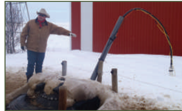
Chad Ross explains his winter water system: A drilled well, submersible pump, arcing hose into a mine tire trough with rubber drinking tubes.
