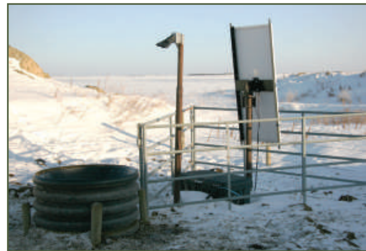
Drain-back solar powered winter water system. A wet well installed beside a large dugout, housed by an insulated culvert provides winter water for the cattle. The motion sensor detects cattle approaching, which triggers the pump to fill water into the bowl. The dugout in the background is a safe distance away from the wet well, to avoid risk of nutrient run-off back into the source water. To protect dugout water further, the pipe is angled downwards into the wet well from the dugout as to prevent water from draining back into the dugout.
