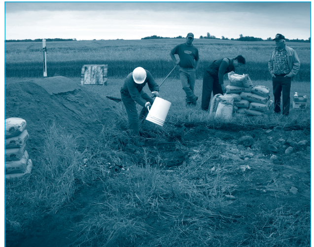
Abandoned water well decommissioning workshop
